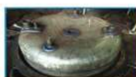
Gas Carburising Furnace
