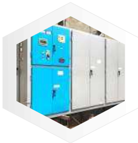
INDUCTION MELTING FURNACE
