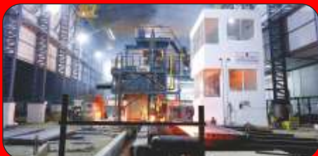
Continuous Casting Machine
