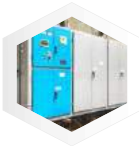
INDUCTION MELTING FURNACE
